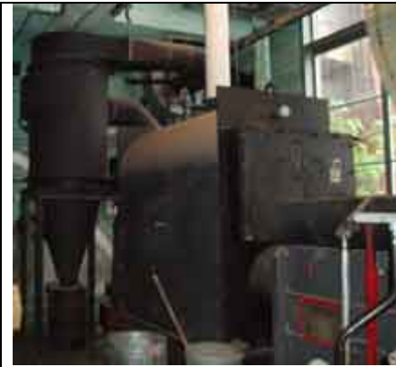
1. 3 MMBtuh Boiler with Gasifier, MA
