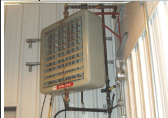
21. Air Heater in Sanitary Plant
