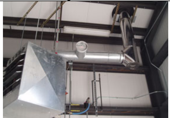
10. Heater and Stack (1 of 2)
