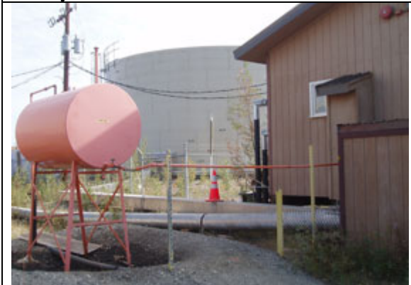
21. Fuel Oil, Hot Water, Water Supply
