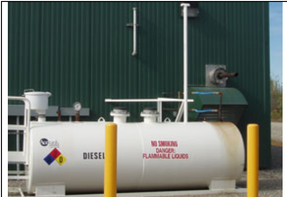
7. Diesel storage, Engine Exhaust
