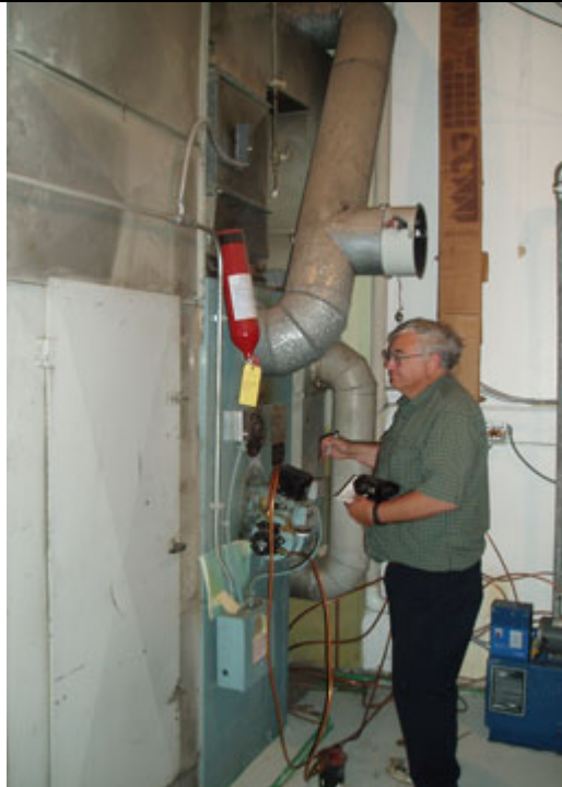
10. Oil fired Air Heater
