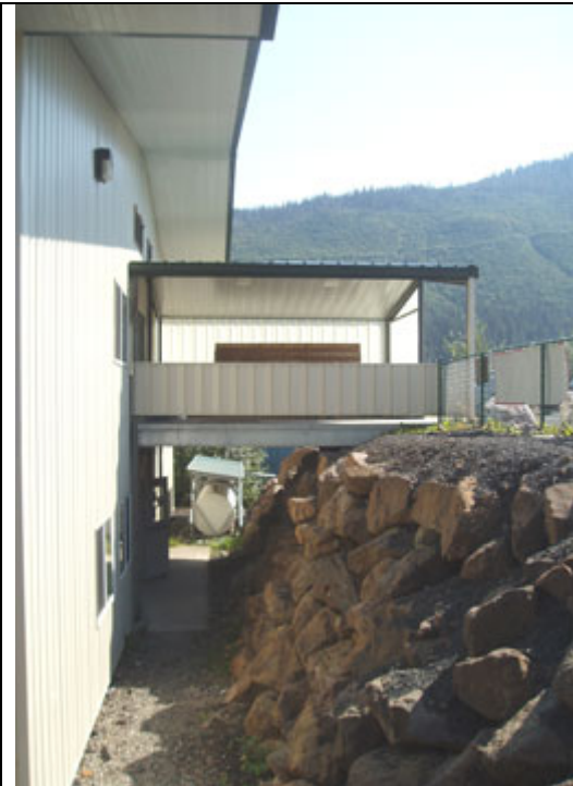
7. Bridge Entry. Fuel Oil Tank Near Boiler
