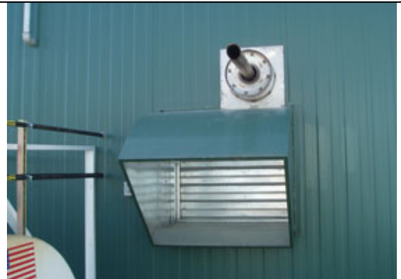
8. Heat Vent and Engine Exhaust
