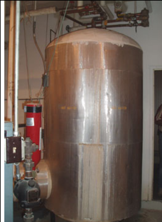
9. Hot Water Heater
