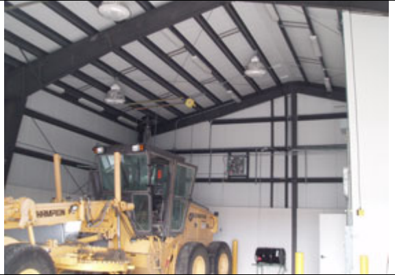
11. Heated Equipment Room
