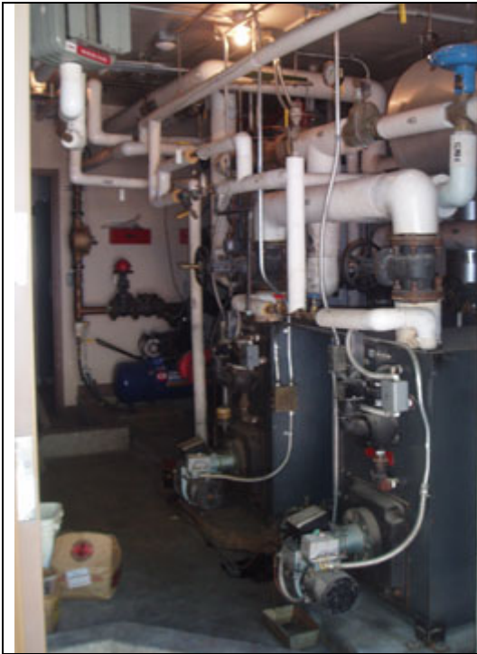
7. Boilers in Upper Building
