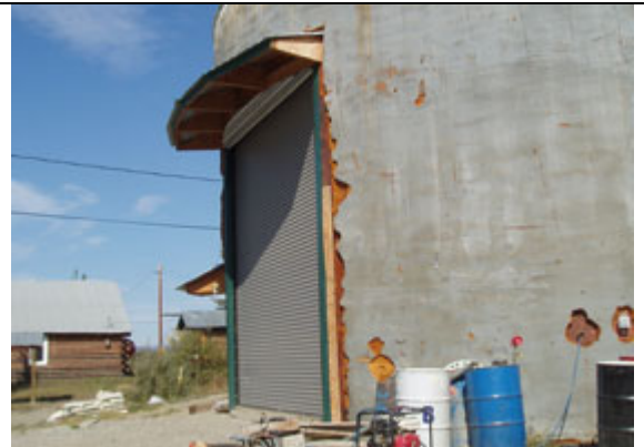
22. Shop: Converted Water Tank
