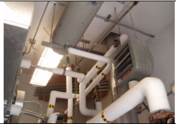
14. Duct Exchanger and Unit Heater
