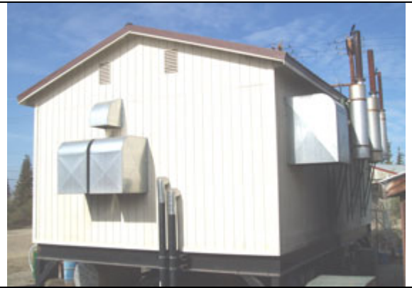
20. Hot Water From Generator Exhaust
