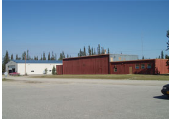
13. Vocational Tech and Buildings
