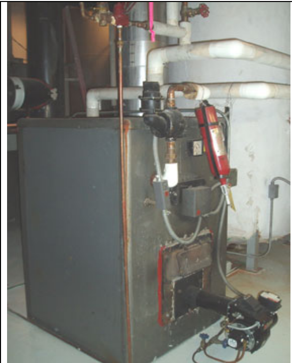
7. Typical Oil Boiler
