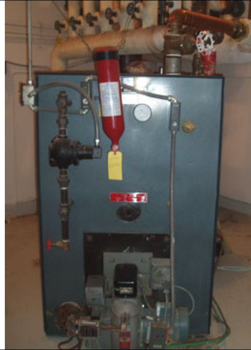
12. Boiler at High School
