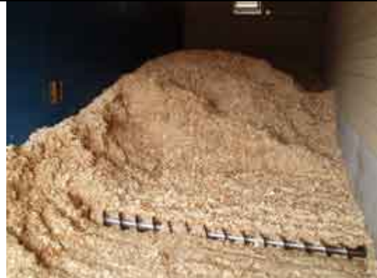
4. Fuel Bin With Chip Reclaim Auger, Victor MT
