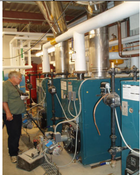
22. 4 MMBtuh (3 Boilers)+ Hot Water
