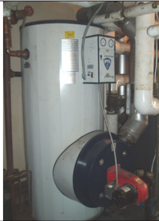
8. Water Heater Upper Building
