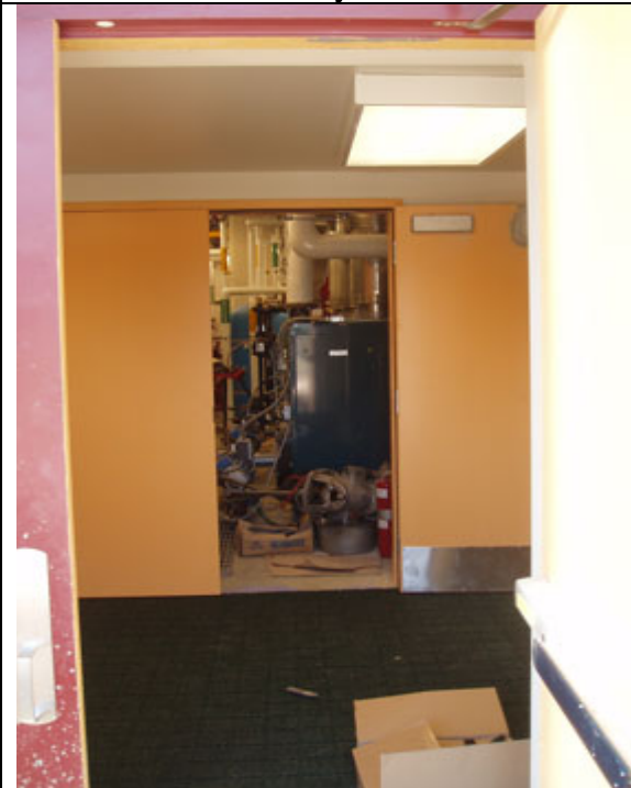
21. New Elementary Boiler Room
