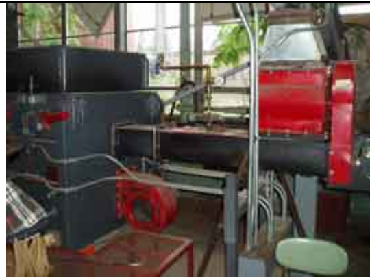
2. 3 MMBtuh Chiptek Gasifier, Athol, MA
