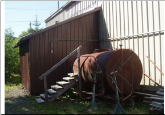
13. Fuel Oil Tank Near Heater
