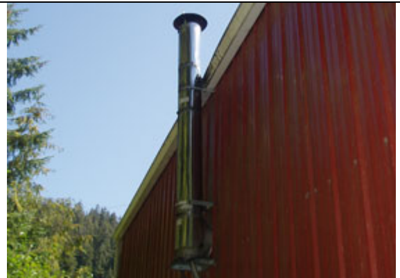
8. Air Heater Exhaust Emergency Services
