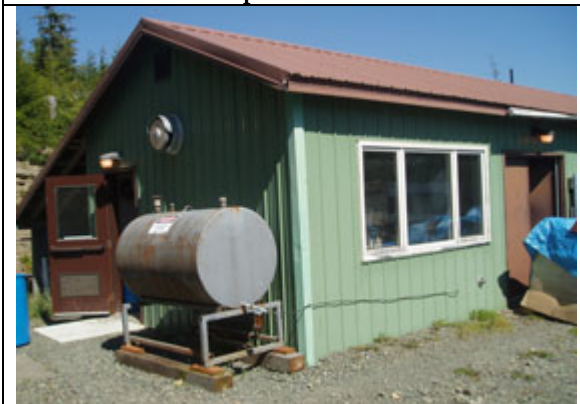
17. Water Treatment South Heater
