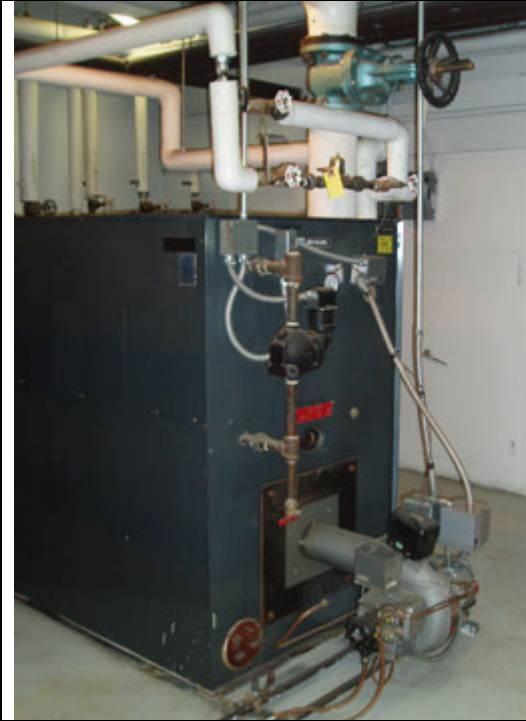
11. Boiler at High School
