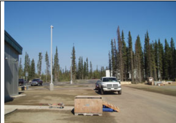
17. View New Elementary to Old Campus
